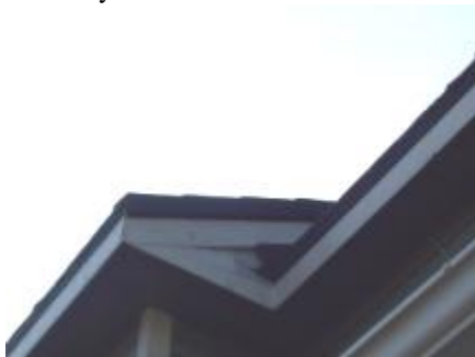
Opening in siding
