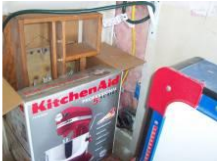
Repair garage drywall
