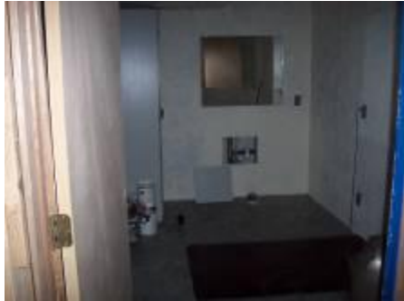
Basement bathroom incomplete
