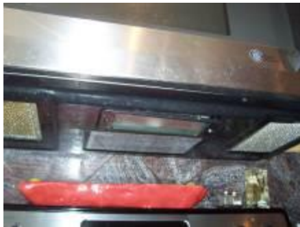
Inoperative microwave light
