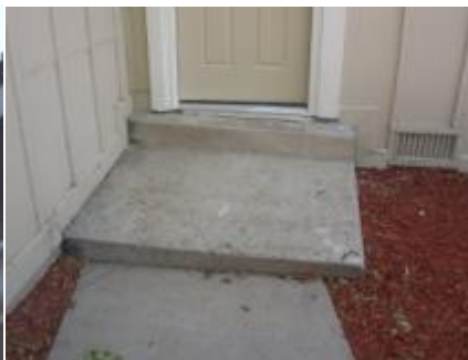
Deteriorated concrete
